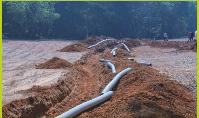
Drainage System works
