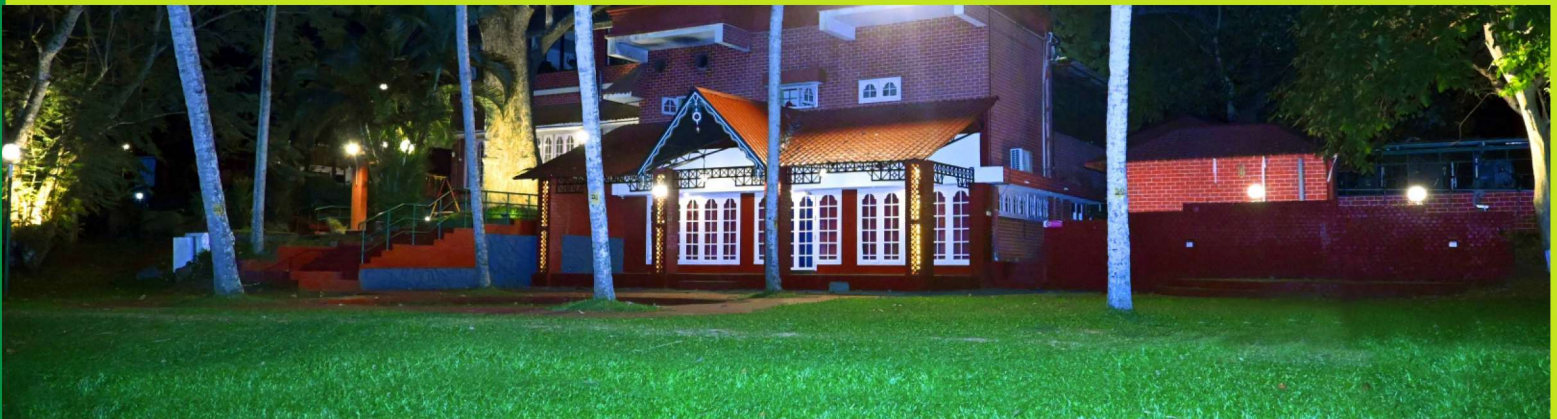
Lawn Area Night View, after installation of New flood Lights
